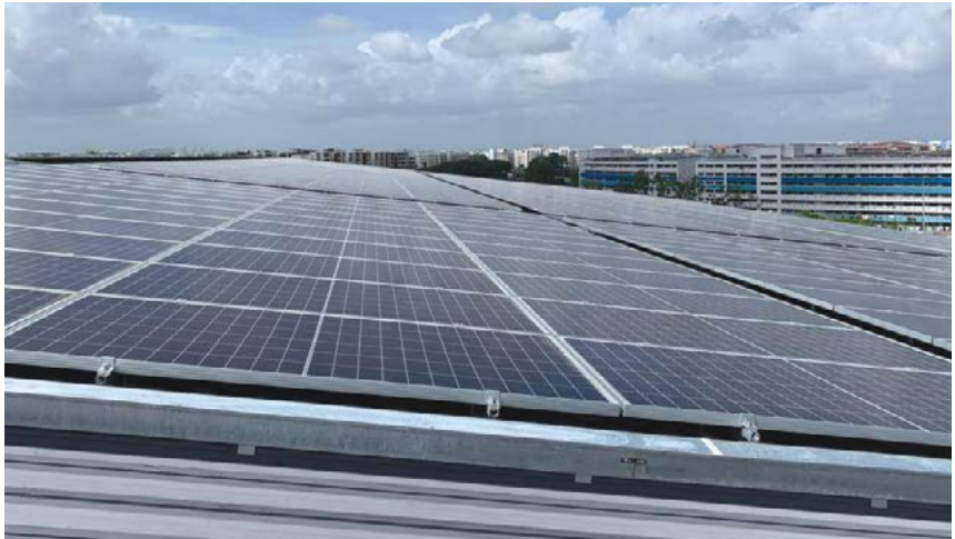
LogisTech is Singapore’s first BCA Green Mark Platinum ‘Super Low Energy’ logistics building.
